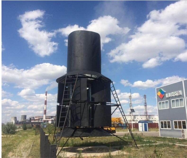
Figure 2-semi-Industrial sample of a vortex wind station.
